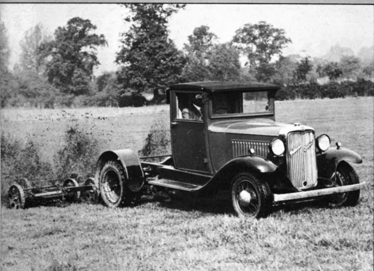
INVENTIVE GENIUS: A Middlesex firm used to convert B-type 12 cwt vans in the 1930s, fit twin rear wheels to them and use them for mowing racecourses, golf courses and the like. The 'bottle' at right,
