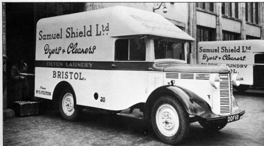
Based on the H-type Vauxhall saloon, the HC 5/6 cwt van (top picture) appeared early in 1938 and was claimed to give 35 mpg fully laden. The 6 cwt Utility Wagon (above) based on the HC was launched in 1939. The larger, 10/12 cwt JC van looked almost exactly like the HC. Two pictures below show some of the main changes made to the W models in mid-1938. Behind the more modern radiator grille sat a more powerful, 72 bhp engine. The radiator filler cap was now out of sight under the bonnet. The 30 cwt WS still sported its original disc wheels; lower picture shows a 3-ton short tipper complete with A.R.P. equipment. Note the difference in bonnet lengths between the 30 cwt and 3-ton models.
